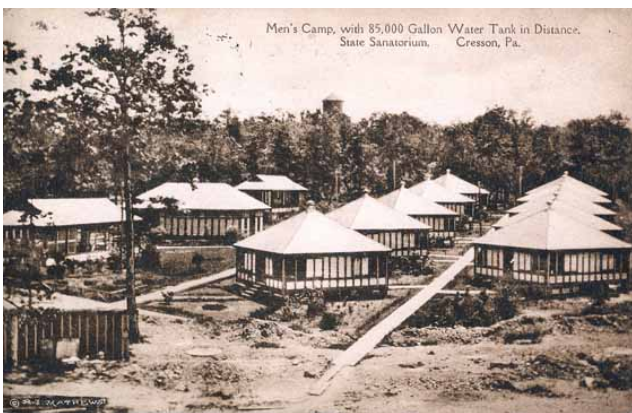
#19 Later photo of Men's Camp with cement sidewalks being installed. It shows the 85,000 gallon water tank in the background.
