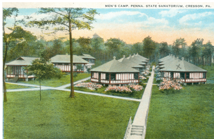
#20.5 Men's Cottages with sidewalks and landscaping complete.
