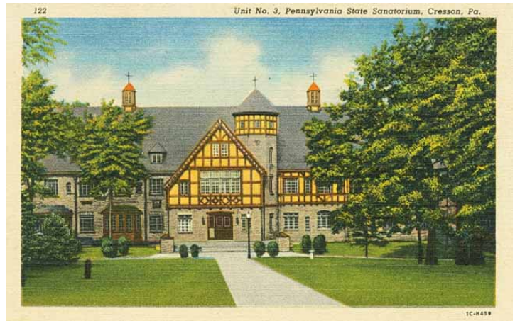
#30 Children's House was opened in 1932. However, the children's department was discontinued in 1950 and it became Unit 3, a hospital building for adults.
