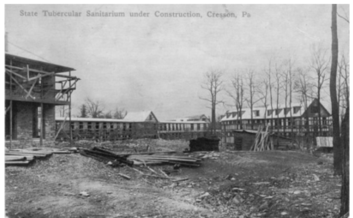
#12 East Wing and Corridor under construction (same view as photo #11). This is the only construction photo of the san I have been able to find. Mailed in 1912 to Hollidaysburg, Pa.
