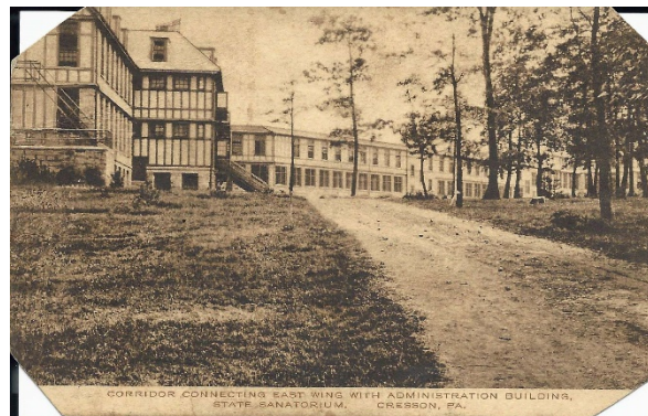
#14.5 East Wing Corridor.
