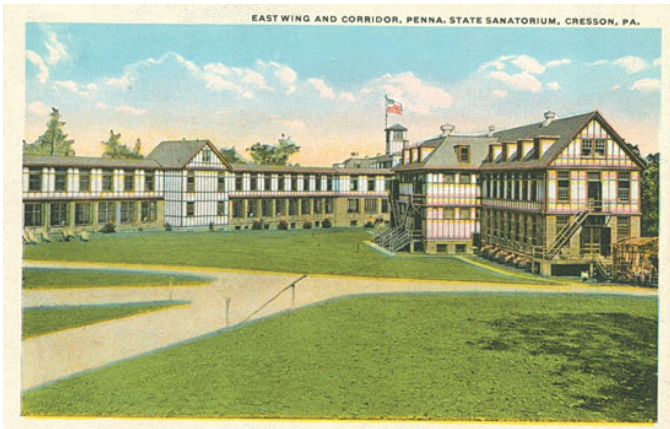
#11 East Wing and Corridor as seen from the back side of photo #10.
