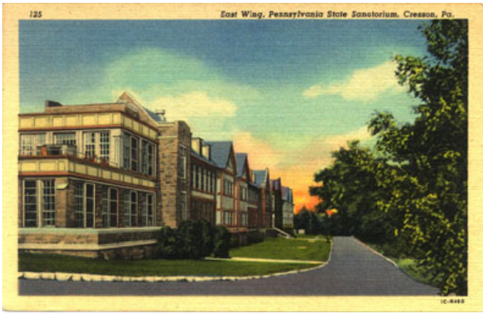
#13 Women's East Wing. Sunroom and sun porch additions on the end of the original building built in 1918. Compare with #9.
