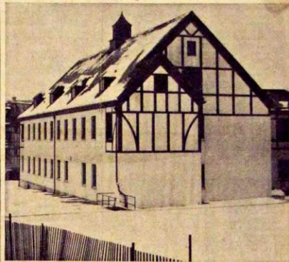
The new $400,000 three-story wing of the State Sanatorium on Cresson Mountain has been opened. Containing more than 5,000 square feet of space, it is known as the medical service building. The latest equipment used in diagnosis has been installed. The building contains beds for 34 patients in 17 rooms, an X-ray laboratory, a laboratory where all manner of tests including microscopic and blood examinations are made, a complete pharmacy, room for consultants to make examinations and give service and a dental clinic. The new facility will aid greatly in enabling the sanatorium staff specialists to speed diagnosis of patients. It adjoins the main hospital structure.
